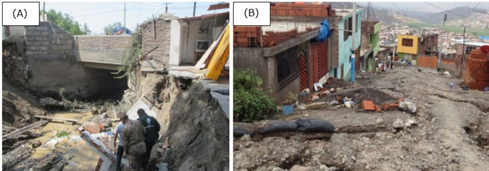
Figure 8. Record of March 8 and January 30, 2017. A) Collapse of the Concordia Bridge in the Chulo stream due to heavy rains that affected the city of Arequipa. B) Heavy rains triggered the activation of the Paucarpata gorge, producing landslides . Source: El Búho (2017a; 2017b)).
