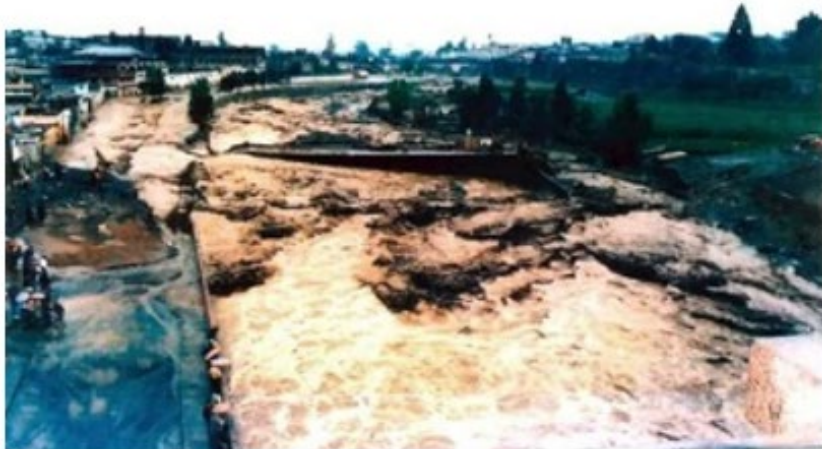
Figure 3. Record of February 8, 1989. A), B) Recorded overflow of the Chili River, as a consequence of the construction of the Bajo Grau bridge that served as a dam, diverting the flow of water through the working-class neighborhood. Source: Climate and Ecology of Arequipa (2013).
