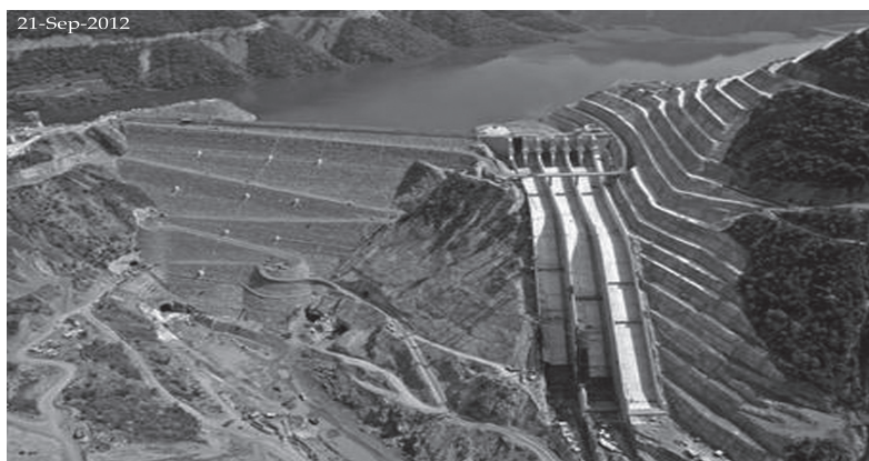
Figure 10. Final spillway conformation (Modified www.cfe.gob.mx ).
