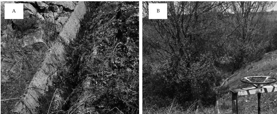
Figure 3. A: Drainage net element of a downstream berm reducing cross-section of water flow. B: Trees rooted behind a service surplus channel downstream of an earth dam.
