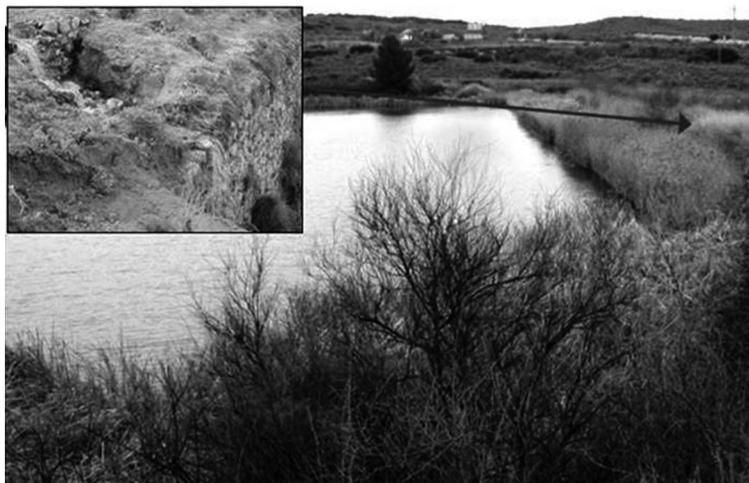
Figure 8. Surface erosion caused by overtopping of a 1552 construction year wall-dam (Ontígola Dam, Spain).
