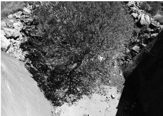
Figure 5. Big tree growing just below the dam crest in the spillway channel of an earth dam, under the spillway dam crest bridge. The channel continues with a rip-rap cover along the downstream slope.
